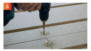
ProFloor boards should be screwed to the base with screws suitable for screwing wood. The screws should be countersunk screws 50-75mm in length. The screws are attached to the middle and the edges of the boards 300-450mm apart.
