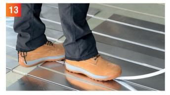
Install the heating pipes into the grooves of the heat transfer plates. Make sure, that the pipe is fully embedded to the groove to avoid it carrying load under the final floor surface. To ensure the pipe sits flat into the groove, lay the coil of the pipe flat to the floor
