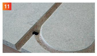
The inlets are milled before installation of the boards or directly to the floor surface.
