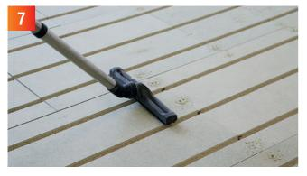
Before installing the heat transfer plates, the floor and the piping grooves should be cleaned of sawdust and other dirt.
