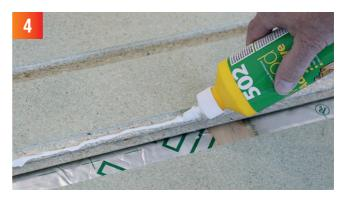
The boards should always be glued to each other at the tongue and the groove. The boards can also be glued to the base to avoid possible creaking. The glue should be an appropriate PVA wood glue. Application of the glue should be done carefully ensuring that there is a continuous seam of adhesive along the entire length of the tongue and groove. Note however that excessive use of glue might lead to gaps between the boards.
