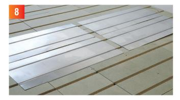
The heat transfer plates are installed by pressing them to the straight sections of ProFloor boards. The distance between the heat transfer plates has to be 10-100mm. There is no need to attach the heat transfer plates to the base.
