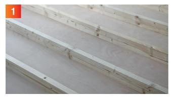
ProFloor boards should be installed perpendicular onto the joists or battens. The joist or batten centres must be no greater than 400mm. In circumstances where the joists are further apart, additional battening should be installed and spaced accordingly. For spaced boarding a minimum of 22 & 100mm boards should be used. For further information please call our technical team on 01268 567019 or consult a structural engineer.
