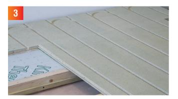
It is recommended to start installation at the furthest place from the water manifold to enable easy installation of the transfer pipes between the piping and the manifold.
