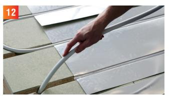
The installation of the heating pipe is begun by passing it through the floor to the manifold
