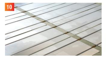
70-90% of the floor area should be covered by the heat transfer plates. The floor should be cleaned once more before the installation of the pipework.
