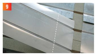
Cut the plates to the correct size. Straighten any bent corners of the plates before installation.
